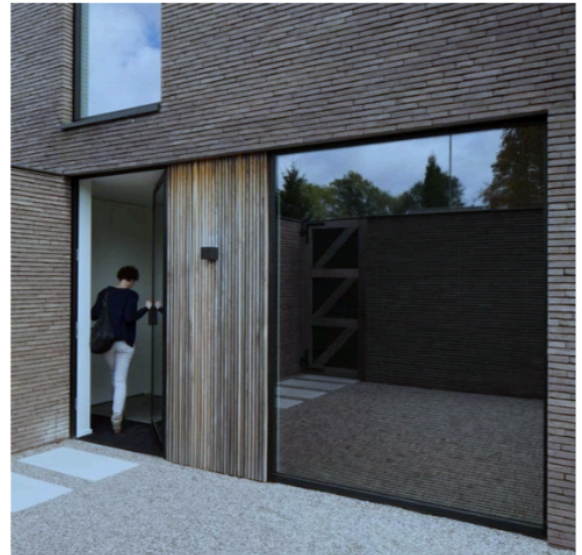
Entrance identified through material change/ expansive glazing
